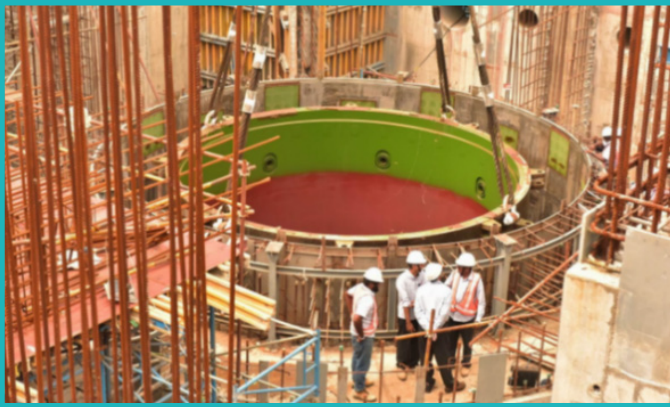
Core Catcher Erection in KKNPP-3
