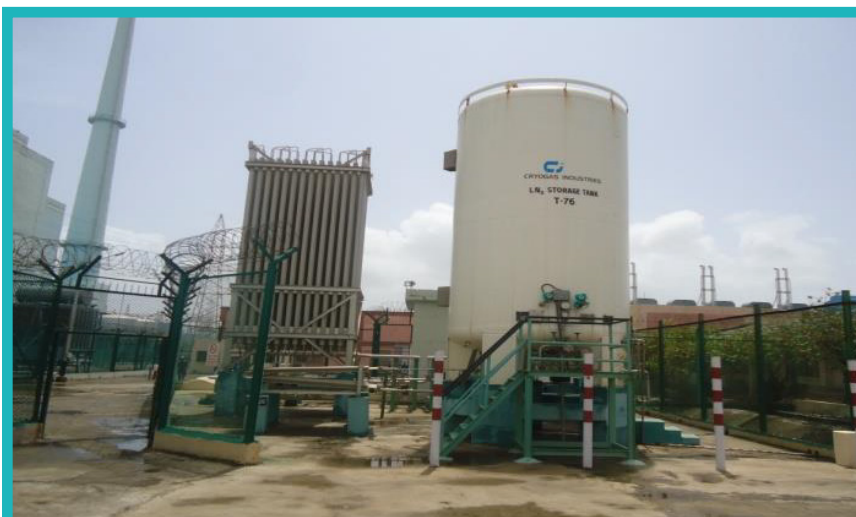
Nitrogen Inerting System at TAPS-1&2
