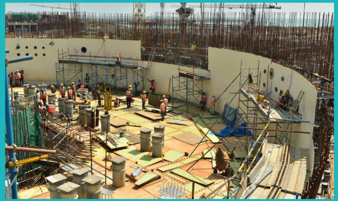
Liner Erection Works in Reactor Building of KKNPP-4
