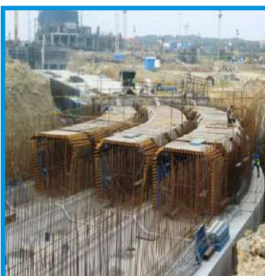
Under Construction Intake Tunnels
