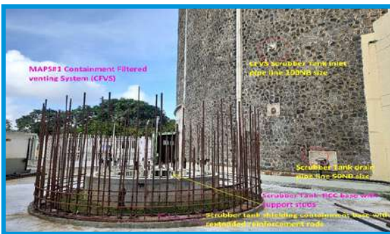
CFVS Construction at MAPS-1&2
