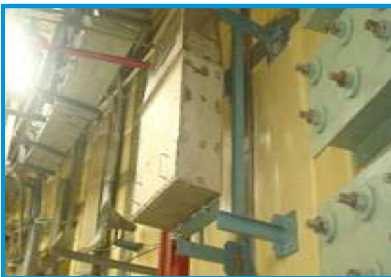
PCRDs installed at RAPS-3&4
