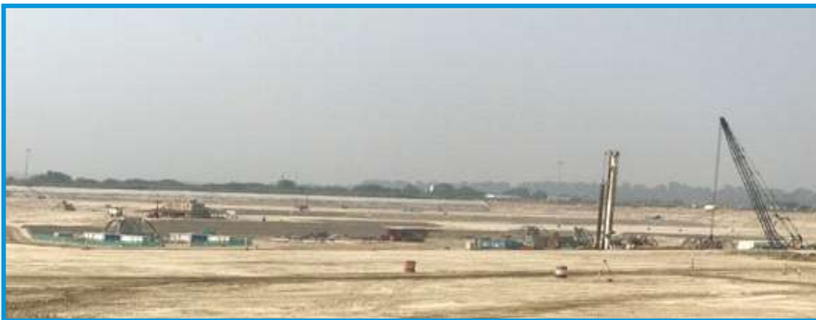
GHAVP-1&2 Site ready for First Pour of Concrete after Excavation
