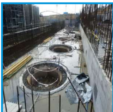
Under construction Main Pump-house
