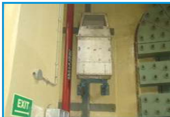
PCRDs installed at RAPS-3&4
