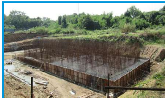
Construction of OESC at Kakrapar, Gujarat site
