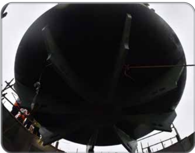
Core Catcher Installation in KKNPP-5
