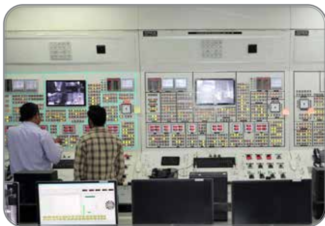
Fuel Handling Control Panel of KAPP-3
