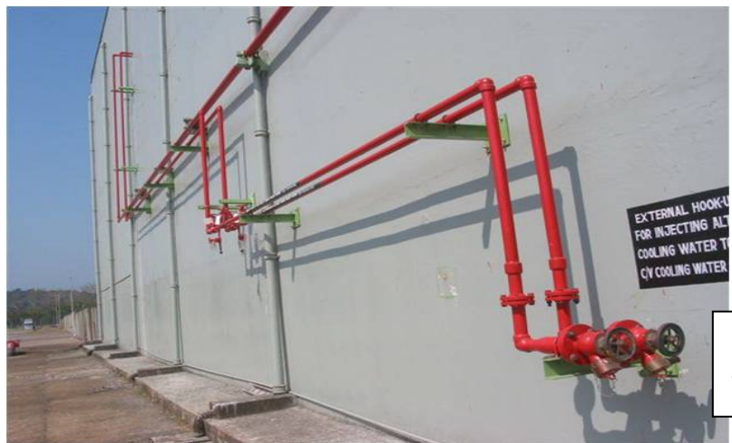
External Hookup points for addition of water to Reactor systems
