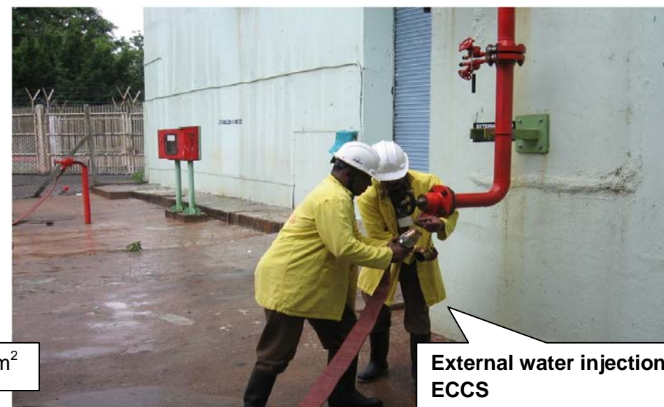
Mock exercise for checking adequacy of mobile pump with the hookup points at KGS-1&2
