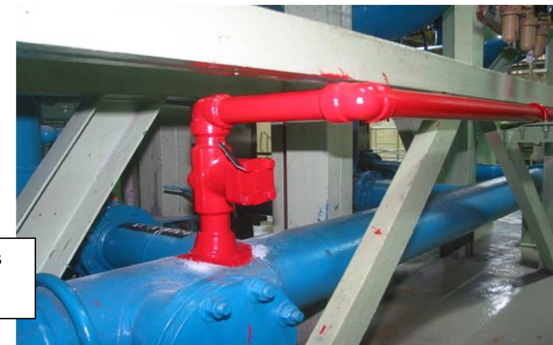
External Hookup points for addition of water to Reactor systems
