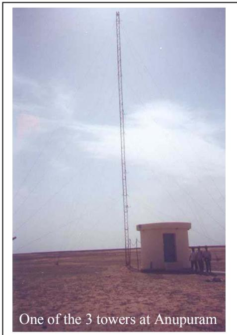
The tower was instrumented with 3 cup anemometers and direction sensors at 10m, 17m, 29m and 50m respectively to study the wind characteristics. For measurement of wind induced tower
