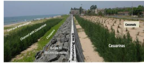
Fig. 6 : Typical elements of Tsunami Protection Wall constructed along Kalpakkam Township
