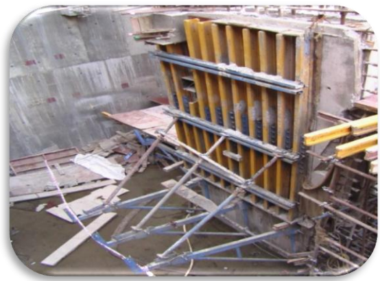
H-Form work shuttering on the wall
