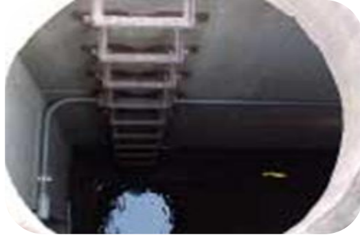
Confined space with safe arrangement for access and egress
