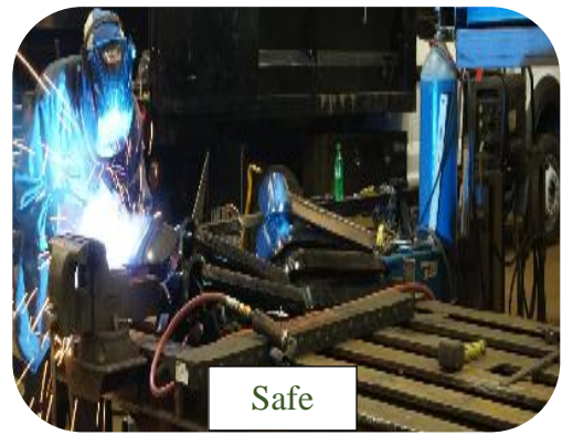
Gas Cylinder properly placed & worker with proper PPE
