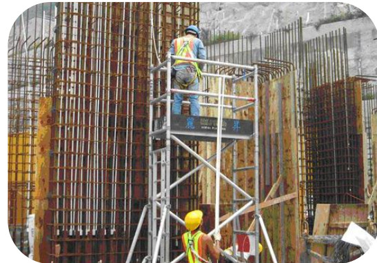
Safe work practice for erection of structure
