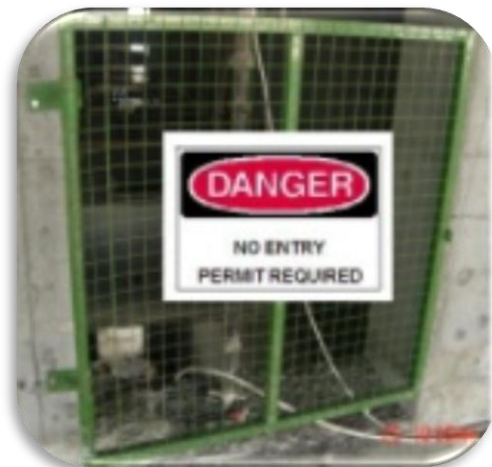
Protection for lift-shaft opening
