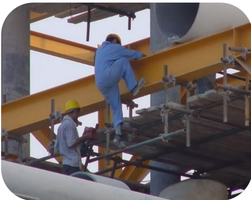
Non-availability of access to higher elevation, compel workers to use wrong practices
