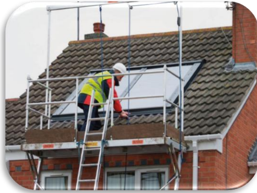
A Ladder for access to height with secure working platform
