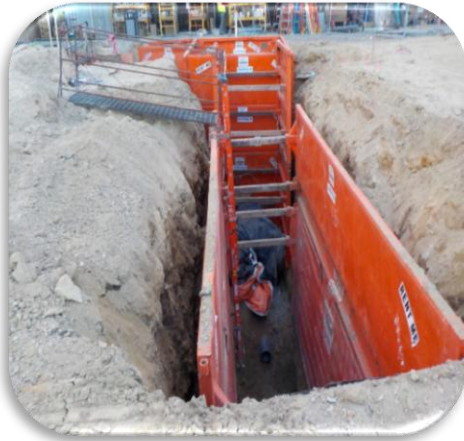
Trench with proper shoring and access
